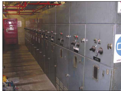
The Rogue's Gallery - typical 25 plus year old switchgear.
